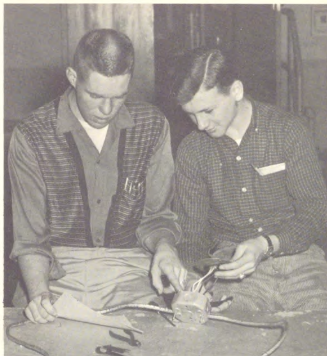
Students Dwight Moody and Larry D. Johnson practice wiring an outlet box.
